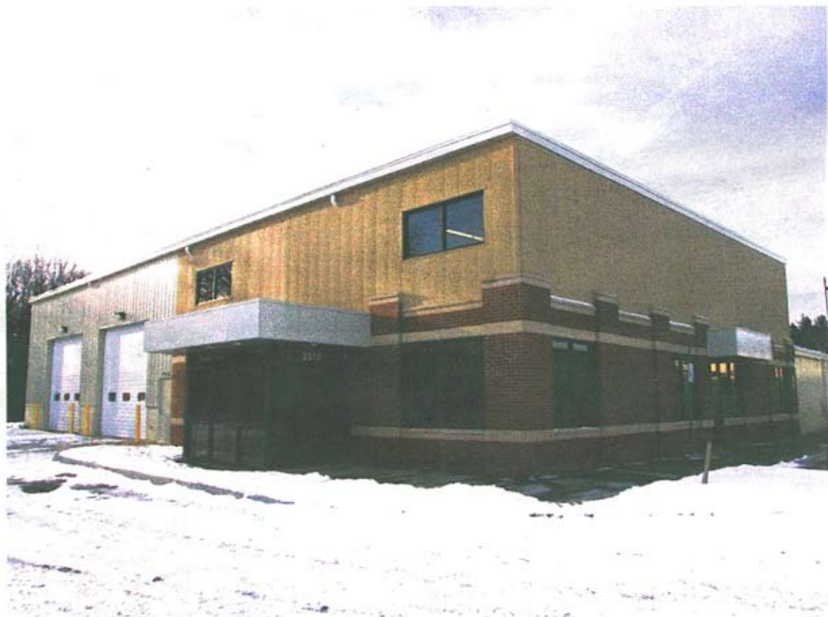
THE EAST GRAND RAPIDS Public Works Complex recently underwent extensive renovation and expansion. Courtesy Wolverine Building Group
